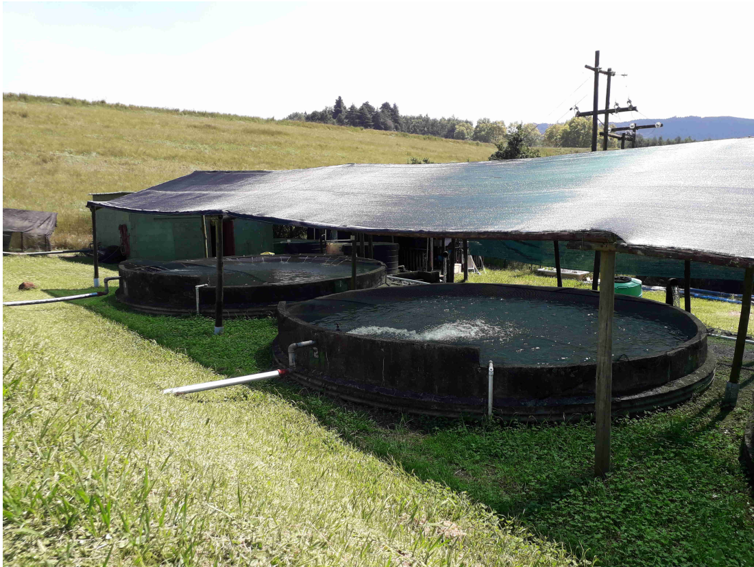
Figure 2.4: Mbona growing ponds are of concrete construction and used for growing the fingerlings to sellable fish of length greater than 6 inches. The flow rate through the pond is controlled by an inlet valve and the depth of water in the tank is determined by the height of the overflow outlet pipe. The ponds are covered with netting to prevent the fish from escaping.
