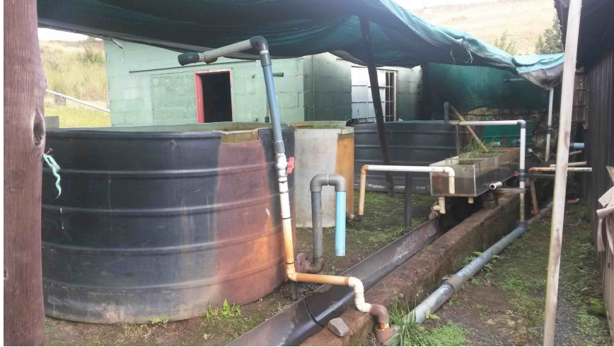
Figure 2.3: Mbona fry tanks are plastic jojo type tanks used for rearing the fry till they are old enough to move to the tanks. The flow rate through the tank is controlled by an inlet valve and the depth of water in the tank is determined by the height of the overflow outlet pipe.
